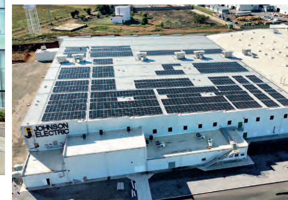
On-site solar panels installed at our Zacatecas, Mexico site are expected to generate 11% of the site’s total electricity consumption
