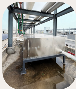
Rooftop installation of a new water storage tank and renovation of pipeline infrastructure to support wastewater reuse
