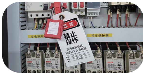
Lock-out/tag-out in Jiangmen, China
