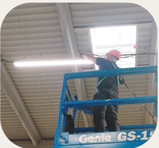
LED light installation at Niš, Serbia
